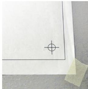
**2.** Use a drill to create one, 3/16" diameter hole through each of the four cross marks. Lightly hammer anchors into each of the four holes.
